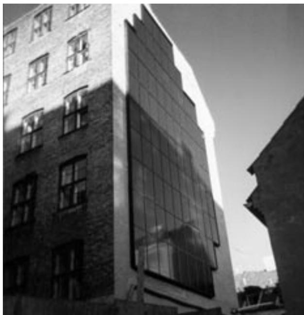
Figure 1. 8.6 kWp crystalline PV-modules from the Danish company Gaia Solar placed on a south facing gable at Viktoriagade 10 B, Vesterbro in Copenhagen.
